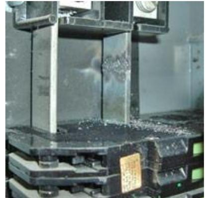
Please, do not attempt to remove breakers from your own panel to see if they've melted. Only licensed electricians should. Zinsco panels can be electrical shock risks; they can appear to be shut off but are still conducting electricity!
